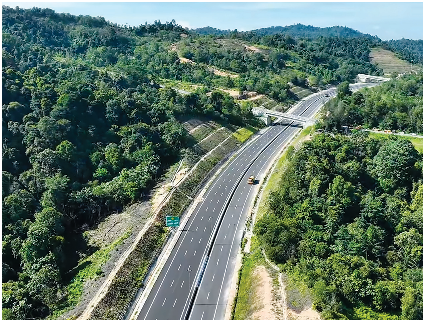
The opening of EKVE Section 1 is anticipated to contribute positively to AZRB's strategic objective.
